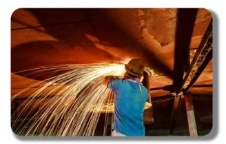
A welder and his helper were attaching tank roof rafters from the tank wall to a roof support center pole. The construction procedure called for them to perform their work at the center pole from inside a manlift basket at a height of approximately 60 feet. Rather than working in the manlift, the workers found it easier to work on a surface attached a few feet below the top of the center pole.
